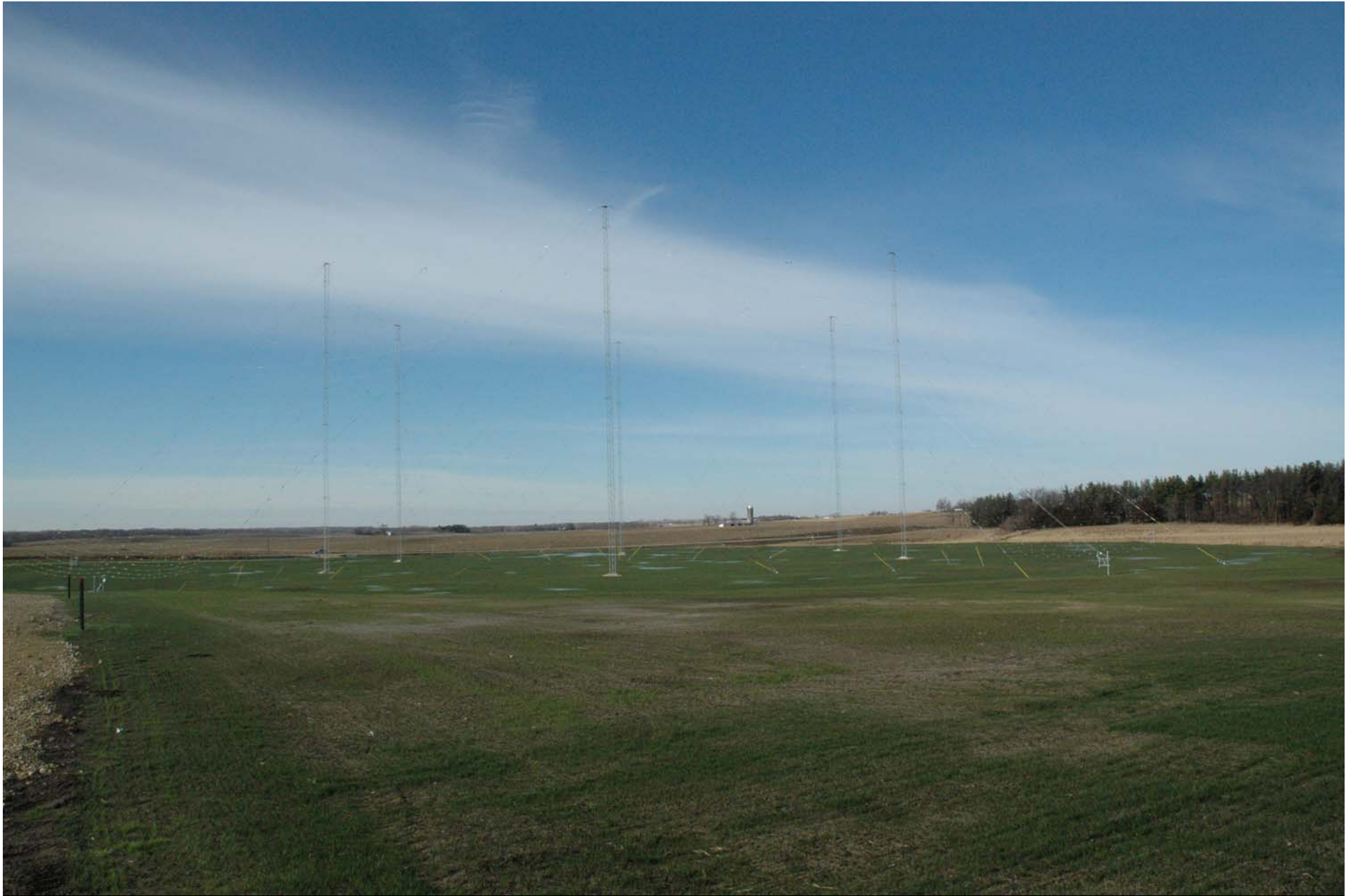
The Array of Six LPH-0406 Log Periodic Curtain Antennas
