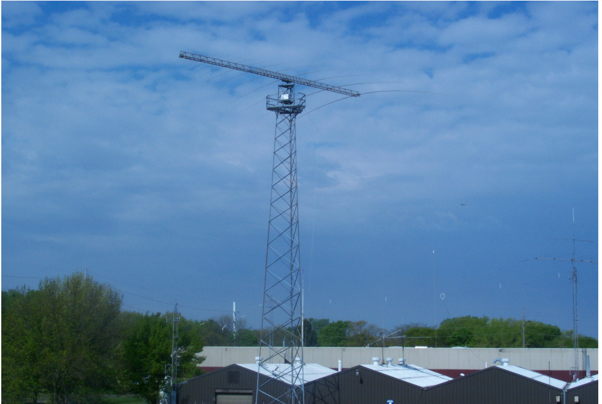
Saber Model 606 RLP Antenna on Self Supporting 100 Foot Tower
