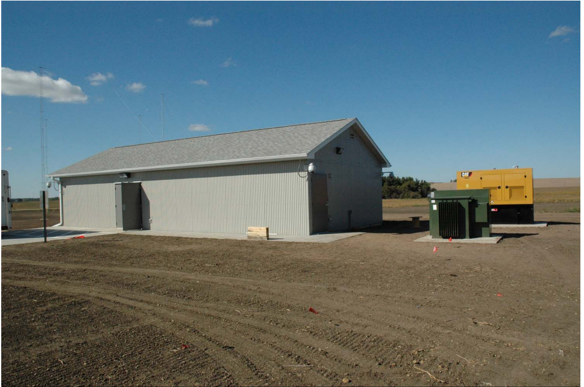
Equipment Building with Emergency Generator
